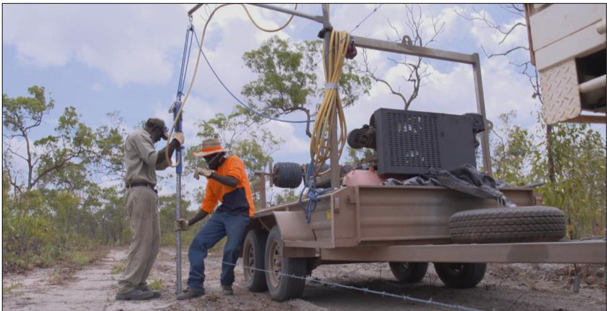
Figure 30: Fence construction (Image from Barber and Creek 2017)
