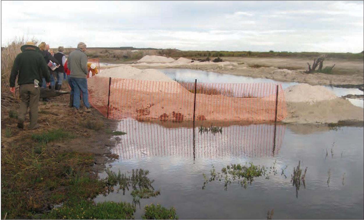
Figure 2.9.10 Applications of fine limestone in the Finnis River below Wally's Landing jetty to acidic waters flowing from the wetland and channel in May 2009. (From Fitzpatrick et al. 2011 d)
