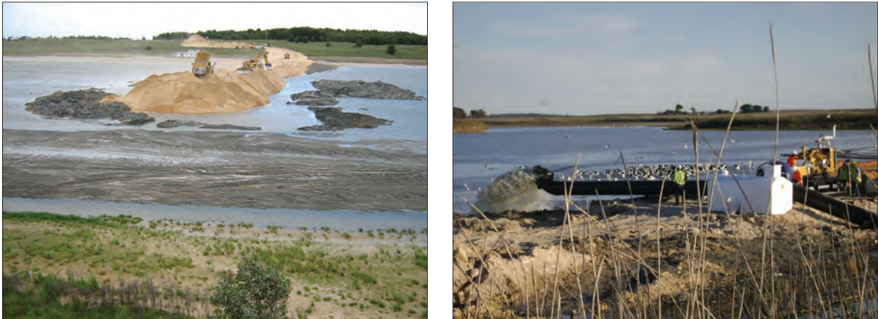
Figure 4.3.3 Temporary embankments to manage acid sulfate soils under construction.
