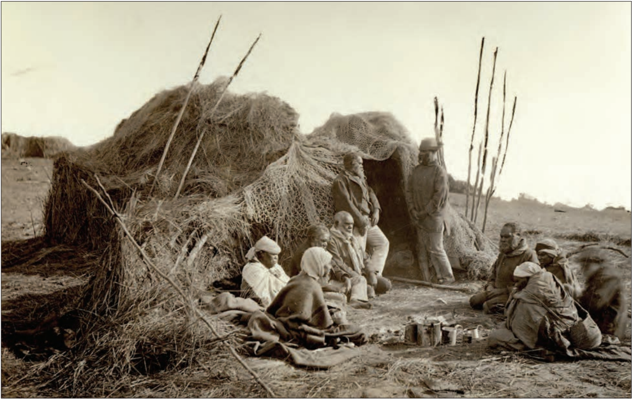
Figure I.1.13 A large Ngarrindjeri ngowanthe (hut) on the hill overlooking Raukkan (Point McLeay Mission) on the shores of Lake Alexandrina in about 1880. The hut is a solid construction, with a timber frame and a windbreak extension. Fishing nets and spears can be seen. (Photographer S. Sweet, courtesy of South Australian Museum)
