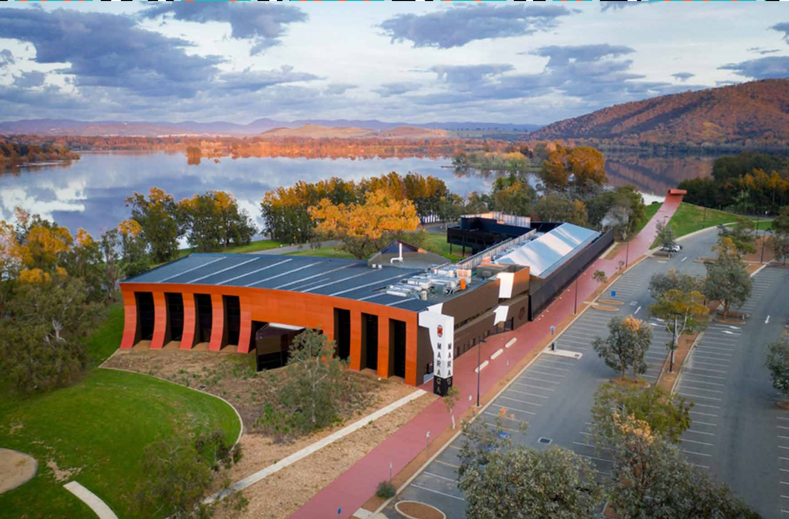
Maraga Building, Ngannawal Country (Canberra), 2021. Photo: AIATSIS
